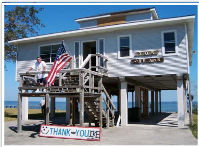
Elevating his home above the Hurricane Ike storm surge saved the house of this Galveston County home owner (FEMA photo).
