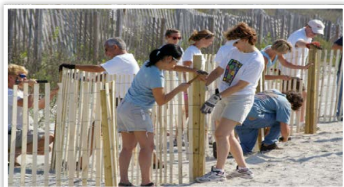
Volunteers install fencing to capture sand and create protective dunes on Folly Beach, SC (Charleston Project Impact).
